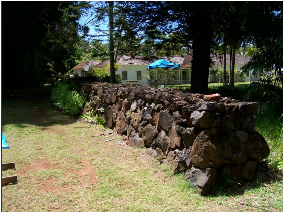
Figure 22: Site 898 Allerton Modification Wall, Overview from the East.
